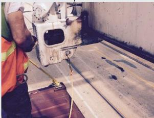
4. Kneel or lay, extend Rescue Pole, Connect Carabiner into D-Ring located on the back of victim's harness and pull the Rescue Pole free. Double check to insure carabiner is securely attached to the victim D-Ring.
